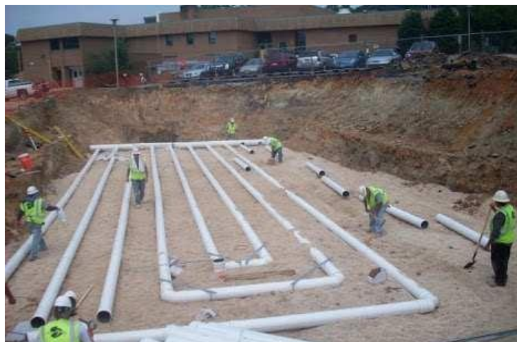
Fig.4 Installation of earth tube
