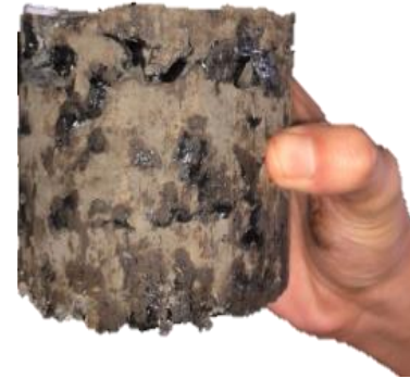
Figure.15 Side view of the CGBM sample obtained. The grout exhibited positive results along with good penetration.
