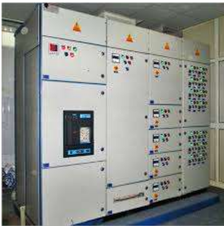
Figure 6 VFD PANEL
